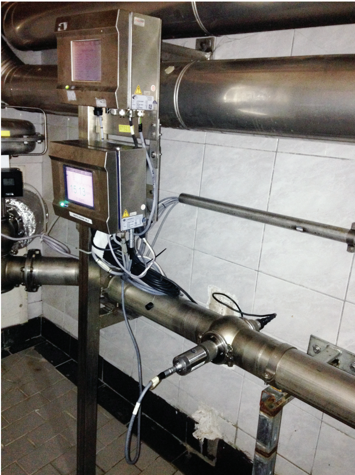
Fig 2. Hach 410 Controllers—typical installation
